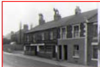
The above image shows the former pub, The Miners Rest at the end of the terrace. On the extreme right is the Spout Lane Pub. Image from raggyspelk.co.uk
